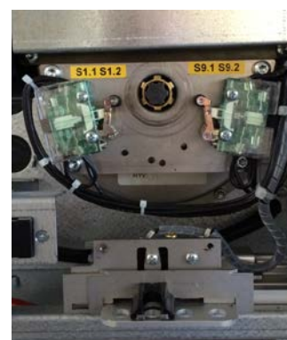
Outer front plate with aux. contacts (picture of UES-K3/10 type)
