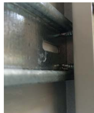
Fixing of installation bar with 4 pcs of 4.2x13 torx-screws
