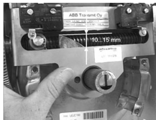
Correct position of lifting arm with operation shaft pushed back
