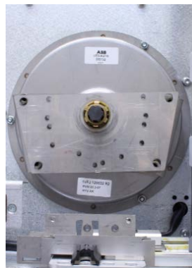
Position indication disc on 1-spring device removed
