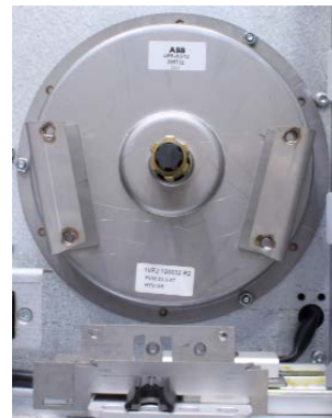
1-spring device without front plates (picture of UES-K3/10 type)
