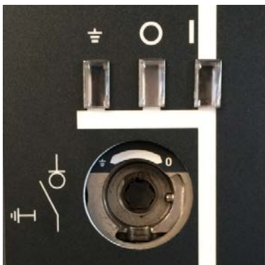
Switch-disconnector in open position
