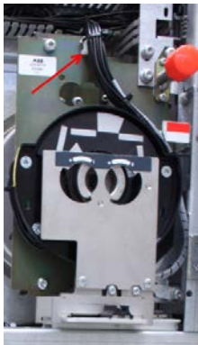
Cable tie on 2-spring device
