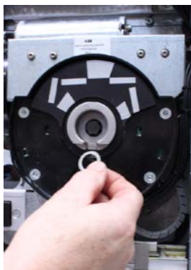
Front position indication disc, operating bushing
