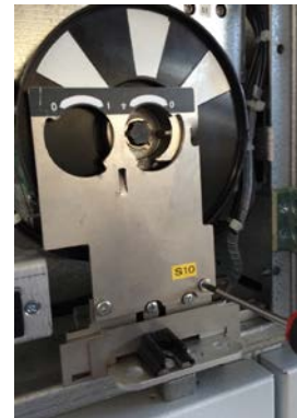
Interlocking front plate installed
