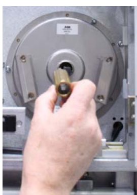
Operation shaft being removed
