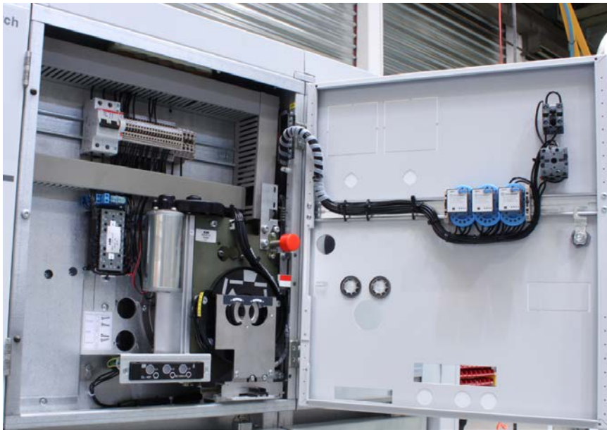
Picture 3.3.1) Example of motor kit for 2-spring device, installed in 500mm wide SDF cubicle.
