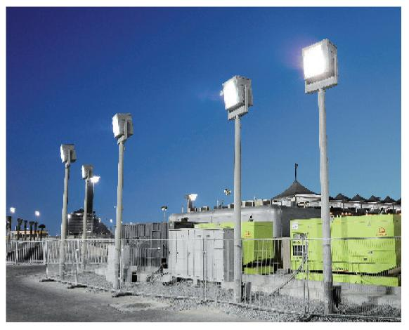
Pramac supplied 44 electricity generators for the lighting system of the Abu Dhabi Formula 1 Grand Prix track. Each one has electrical power from 250 kW to 370 kW and is able to supply enough power to light more than 4,000 flats. Pramac generators are equipped with special anti-sand filters able to prevent any potential blackouts caused by desert sand storms.
