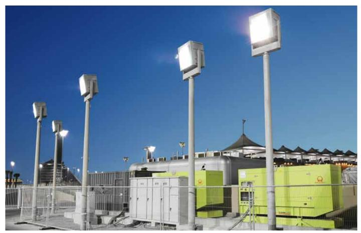
Pramac supplied 44 electricity generators for the lighting system of the Abu Dhabi Formula 1 Grand Prix track. Each one has electrical power from 250 kW to 370 kW and is able to supply enough power to light more than 4,000 flats.
