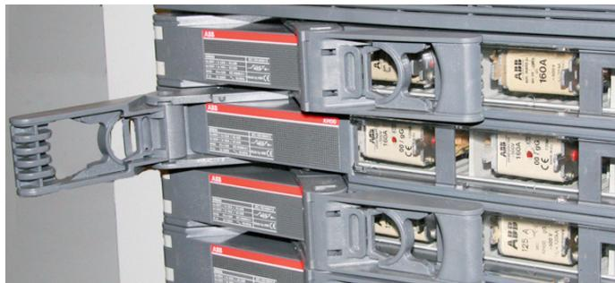
1. Switch OFF the XR where the NH fuses shall be replaced and open the frontcover.
