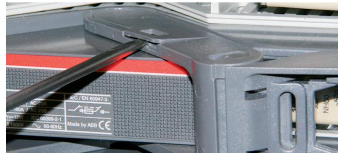
2. The operating handles of the XR's placed above and below can be released by use of a screwdriver and moved to park-position with the XR's still in ON position.
