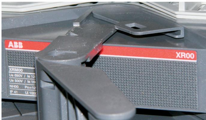
3. With the operating handles above and below in park-position, there is easy access to the L1 fuse in the XR in the middle.
