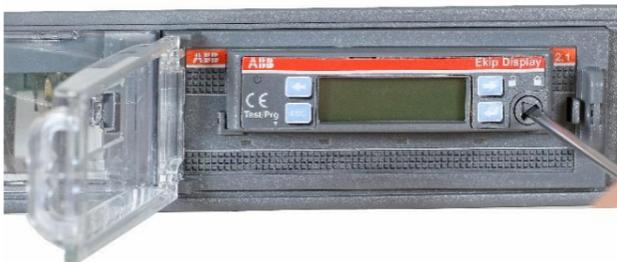
3. Fix the closing button by using a screw driver and rotate to closed position.
