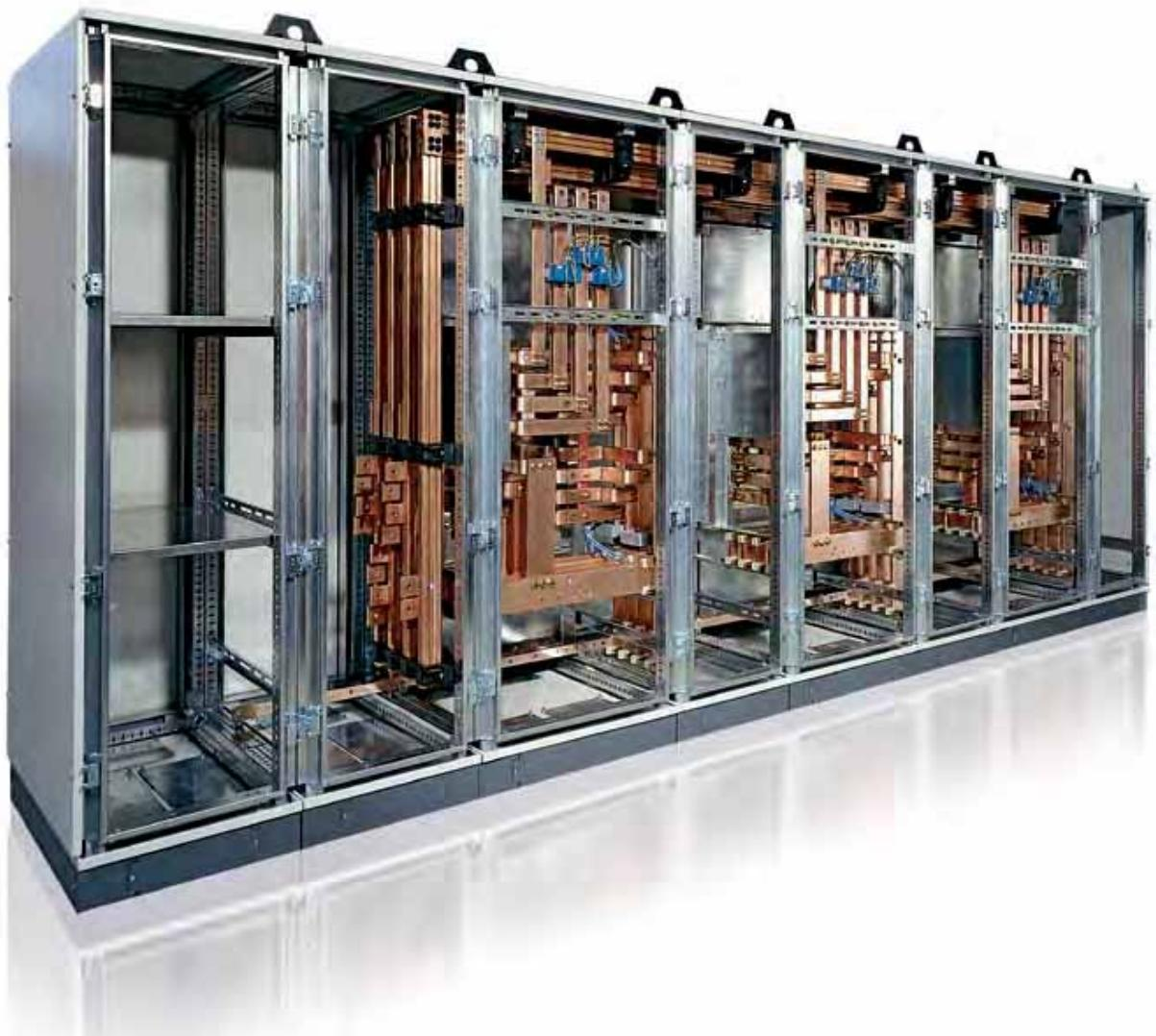
Within the ArTu K series switchgear, like all the series in the range, it is possible to install ABB apparatus (System Pro M modular circuit-breakers, Tmax moulded-case circuit-breakers, T and XT series and Emax air circuit-breakers) with an excellent and certified level of integration. The switchgear is available in four functional widths (390, 600, 800mm and 1000mm) and in two functional heights (1800 and 2000mm), which allow installation of 9 and 10 modules 200mm in height respectively.
