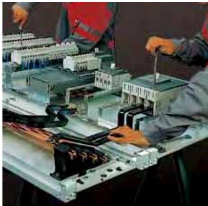
Wiring becomes easier thanks to the completely open structure, and it is in fact possible to wire without problems horizontally on trestles.
