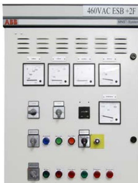
06 Synchronizing Cubicle
