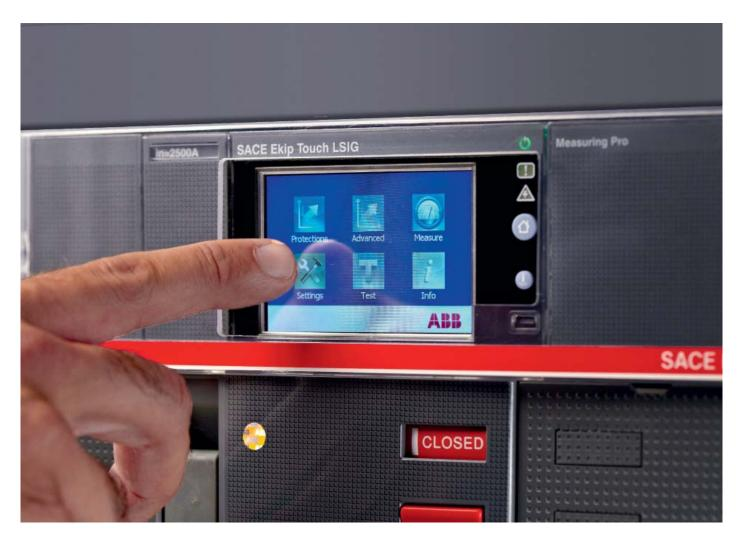
Simplified installation and maintenance. SACE Emax 2 series circuit breakers are equipped with protection trip units containing a large, color touch-screen display for maximum ease of use. Productivity is increased while all stages, from design to daily operations, are simplified.
