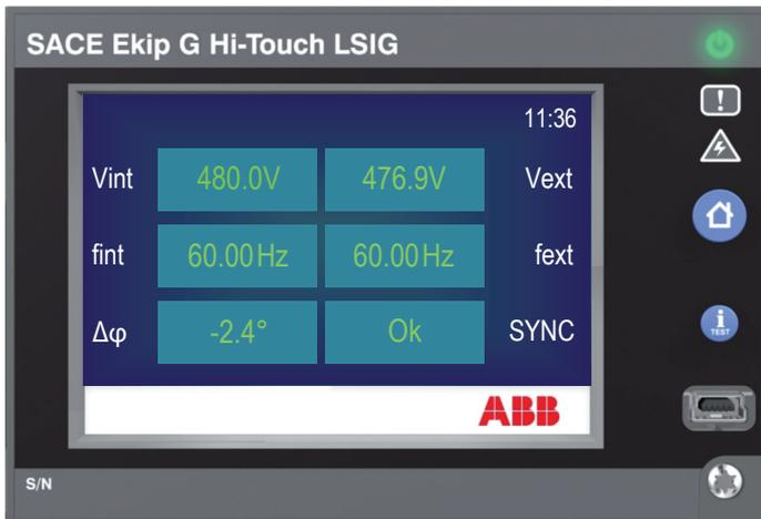
Figure 3 - Ekip Trip Unit Display (in sync)
