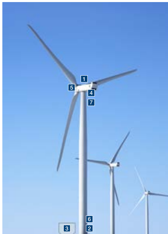
Example on a full converter drive train turbine with power converter installed at the tower base and the LV/MV transformer outside the turbine
