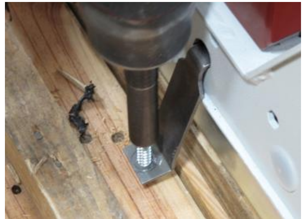
Figure 11: Clamp screws
