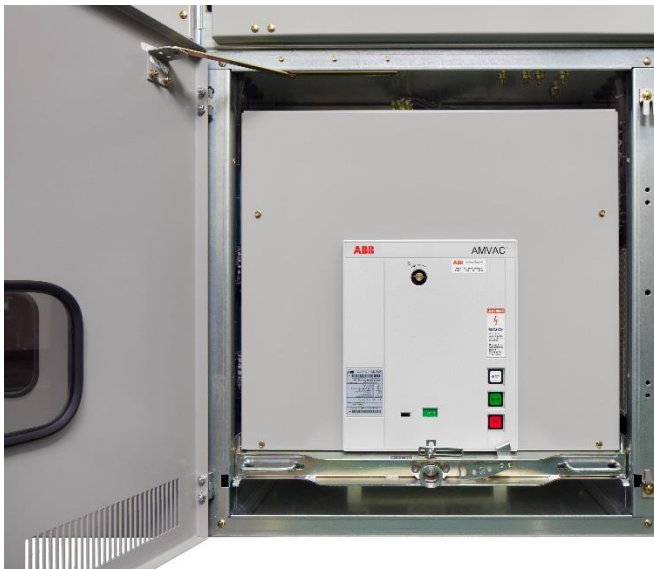
Figure 20: Circuit breaker in DISCONNECT position
