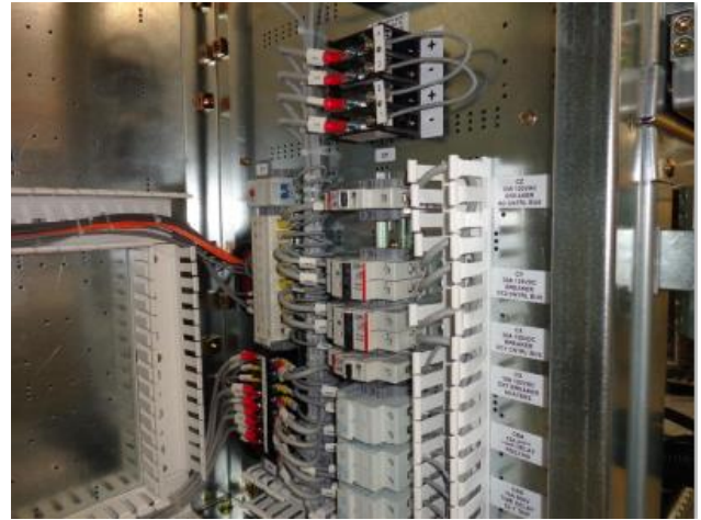
Figure 1: Heater load terminals in low voltage compartment (typ.)
