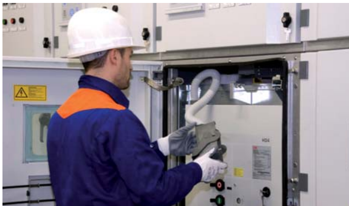
ABB engineer inspecting a circuit breaker during a MySiteCondition assessment
