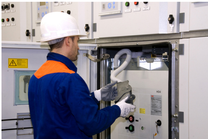
ABB engineer inspecting a circuit breaker during a MySiteCondition assessment
