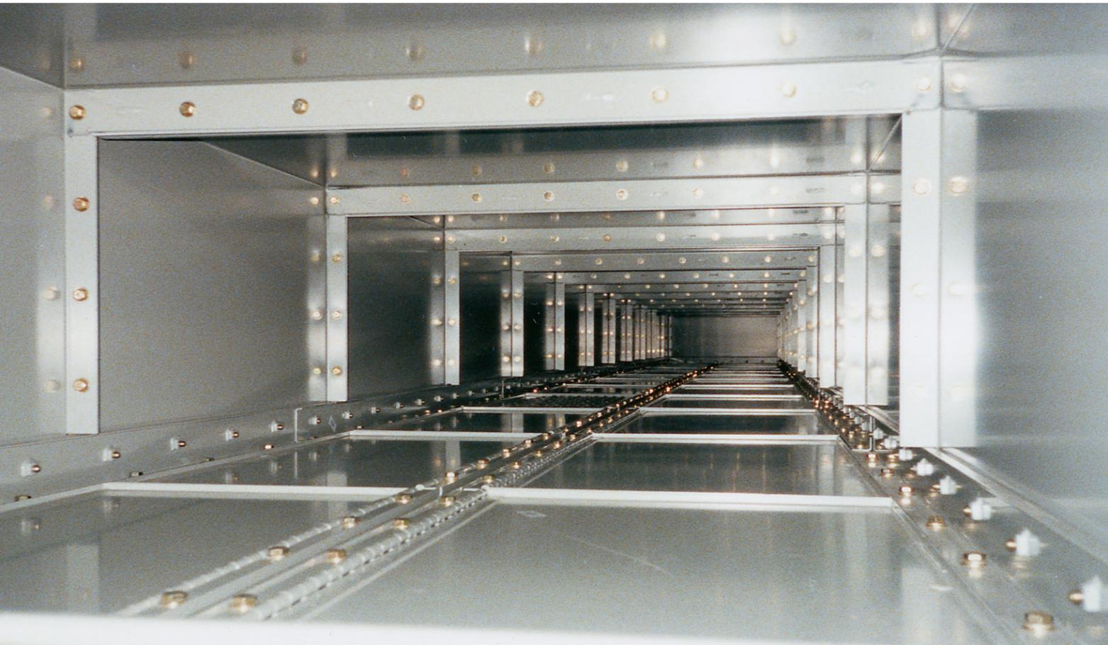
1. Each primary compartment – breakers, auxiliary transformers, main bus, and primary cable entrances – are designed with internal hinged flaps or vents to allow over-pressure and hot gases to escape in a carefully controlled manner through roof mounted plenum exhaust ducts – away from nearby personnel at the front, rear or sides of the switchgear.
