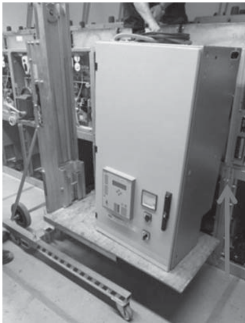
Fig. 2.3.3.3: Examples of lifting the low voltage compartment
