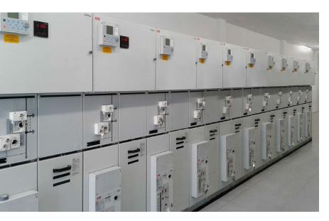
The LC1000 UniSec solution, developed for UniSec medium-voltage switchgear, detects and isolates faults in ring networks within less than 1 second, ensuring a fully functional network and minimized outage time.
