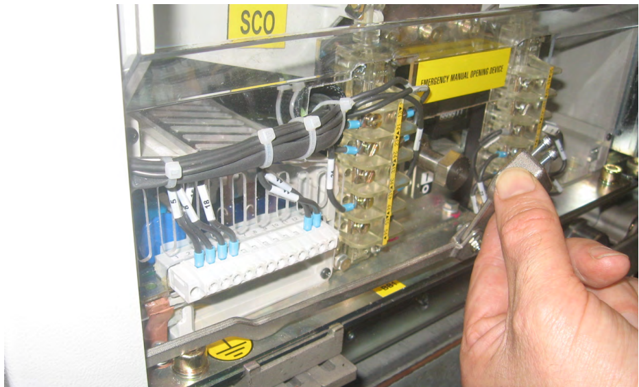
9/7. Mechanical ON/OFF linkage
