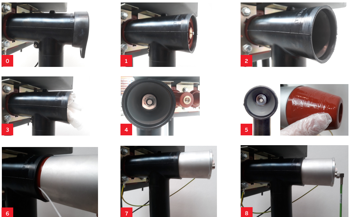
16 KEVA xx C2 4.1(c) sensor mechanical installation
