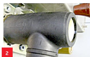
10 KEVA 24 C21(c) sensor mechanical installation
