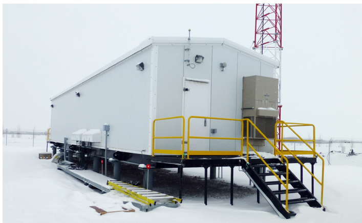
Metal-enclosed electrical houses
