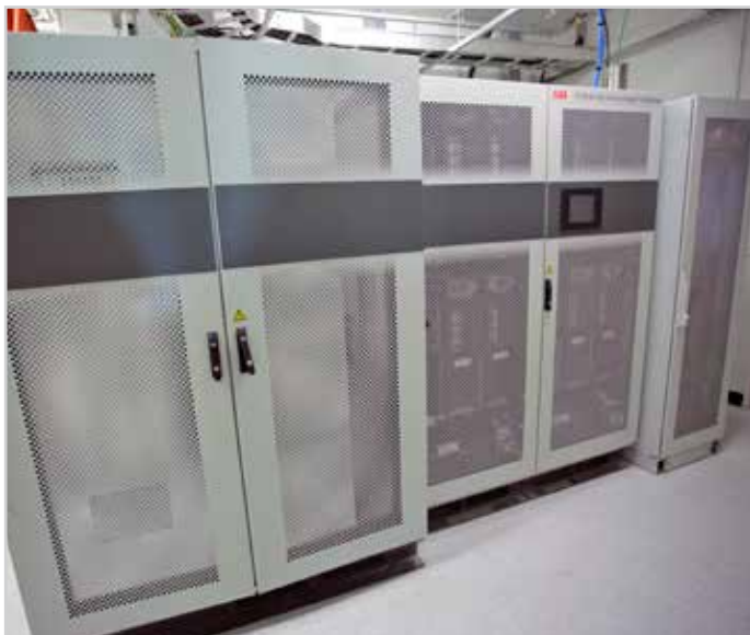
ABB successfully installed a PCS100 Active Voltage Conditioner at Fonterra's facility
