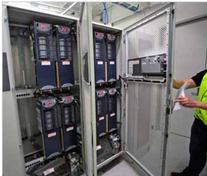
The PCS100 Active Voltage Conditioner has been installed to eliminate voltage sags and correct any power quality problems Fonterra encounters
