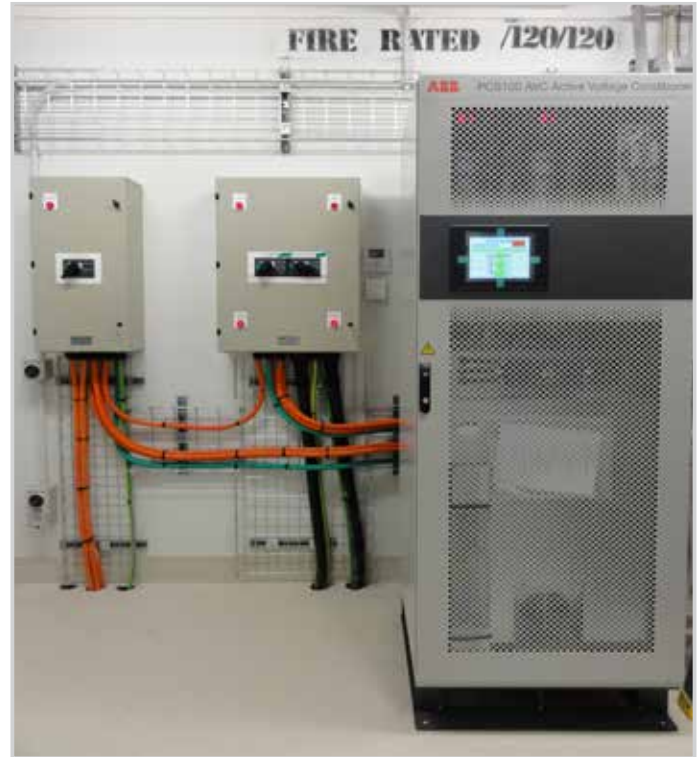
ABB's PCS100 AVC installed at Whakatane Hospital in New Zealand to protect the CT Scanners from suffering a power quality event
