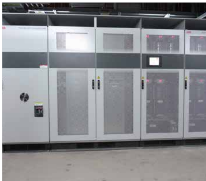
ABB's PCS100 Industrial UPS that has been installed for phase one in Samsung's Suzhou facility to protect against voltage sags
