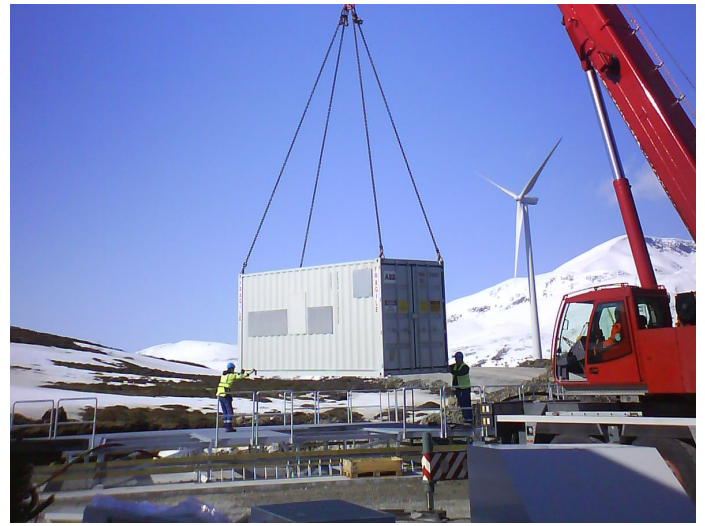
A crane positioning one of the PCS100 STATCOM containers into place
