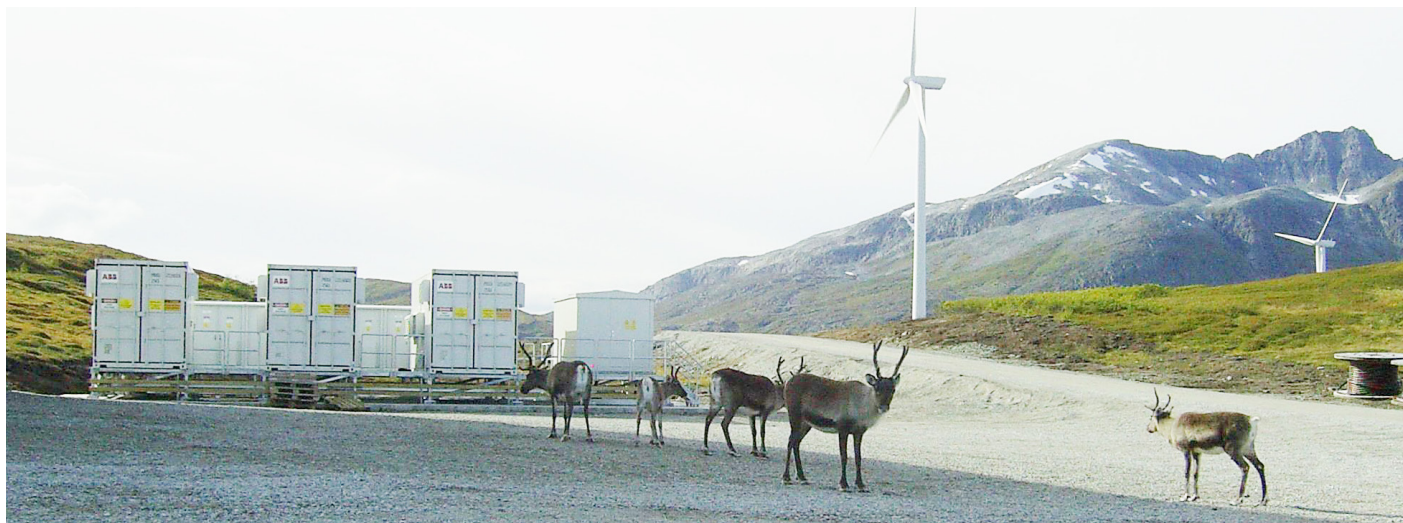
Three 2 MVar PCS100 STATCOM containers for a 54-megawatt onshore wind farm located in Fakken, in the far north of Norway
