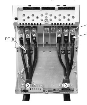
Remove the screw terminals. Fasten the cable lugs to the remaining bolts with M10 nuts.
