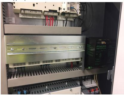
INU APBU when the support plate is removed.
