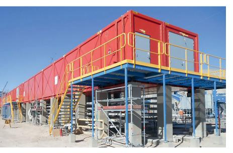
An E-house\* is a modular enclosure housing switchgear, variable speed drives, control systems and substation-related equipment. The flexibility of design means an E-house can be adopted for a wide variety of applications.
