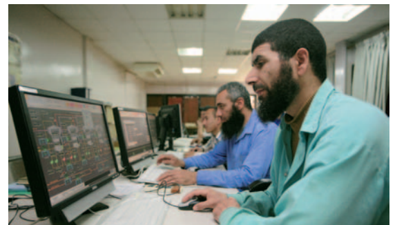
The control room with its System 800xA operator workplaces.
