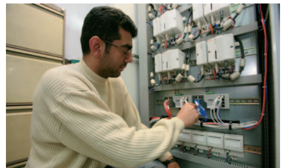
AC 800M controllers in redundant configuration at the sugar plant.
