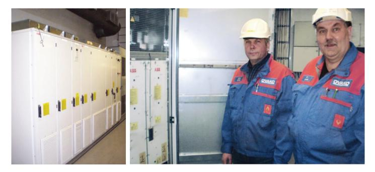
ABB's electromagnetic stirrer for its ladle furnace, LF-EMS, was installed at Ovako Bar Oy Ab in Imatra in southeast Finland in 1988. Production was smooth until 2005 when the old YOQD drive for the stirrer came to the end of its life cycle with three unexpected failures. The old YOQD frequency converter needed to be replaced with ABB's modern ACS 800 drive due to life cycle considerations.
