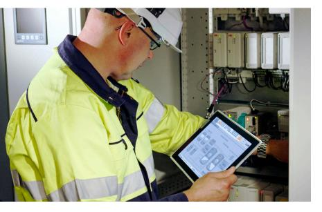
The use of mobile devices in industrial facilities is now widely accepted and can provide tremendous value to day-to-day operations. Utilizing standard technologies, proper network design, and best practices, mobile devices can access the 800xA system over a secure wireless network. Everyone associated with a system can benefit from having immediate access to real-time information.
