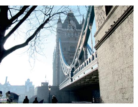
Digital upgrade of ABB load monitoring system helps extend life of London's landmark Tower Bridge. When it was first constructed, Tower Bridge was the largest and most sophisticated bascule bridge ever to be built. The bascules were operated by hydraulics, using steam and giant pumping engines and, despite the complicated procedure, the bascules only took a minute to raise to their maximum angle of 86 degrees.
