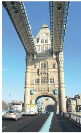
The dead weight of the bascules and the live load of the traffic were not being carried fully on the resting blocks and locking pawls, but also on the shaft bearings. Because of misalignment and wear, the pawls didn't properly lock the ends of the bridge decks in the down position and they didn't correctly engage.
