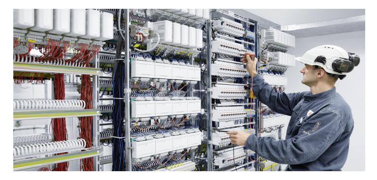
Unsymmetrical current distribution on high power rectifiers results in an accelerated aging process of semiconductors and fuses. The current distribution measurement detects and corrects this.
