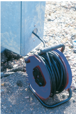
The openings on the sides of the cabinet is used for temporary power outlets, etc.
