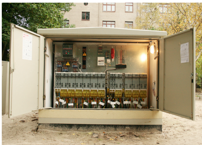
Kabeldon switching devices in a CSS, Latvia.
