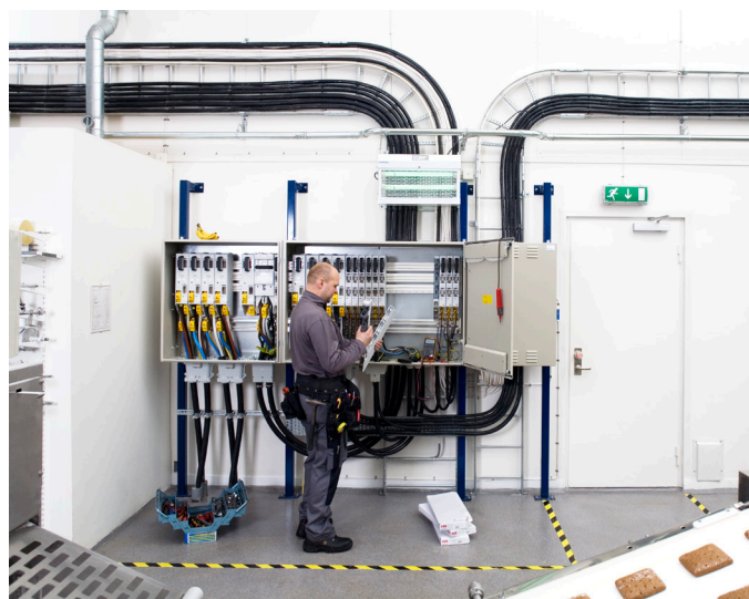
Distribution board in powder coated enclosure mounted on the wall in a switchgear room at a bakery, in Gothenburg, Sweden.
