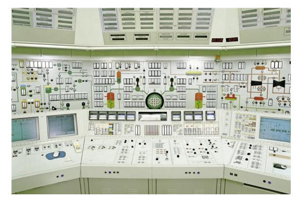
This began to change with digital signals and the distributed control system (DCS) in the 1980s. Panel boards were replaced by monitors and servers, and signals were transmitted from plant equipment to computer processors, where the signals were turned into actionable information.
