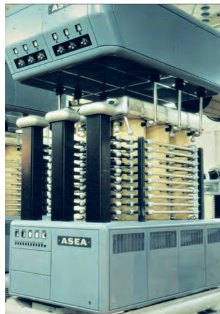
3 Pacific Intertie mercury-arc valve in Sylmar, Los Angeles
