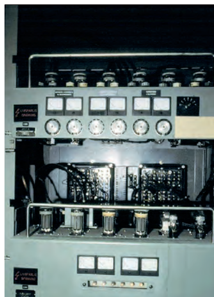
1 Original Gotland converter firing control system based on vacuum tubes
