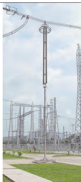
5b 500 kV DC bus arrester (2000)
