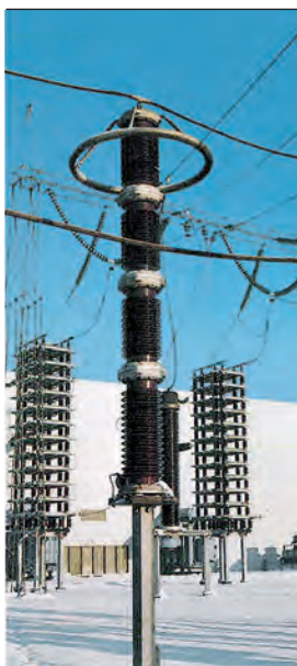
5a Gapless HVDC line arrester (1979)
