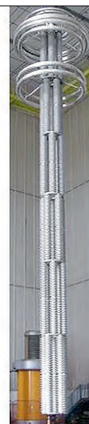
5c 1,100 kV DC bus arrester (2012)
