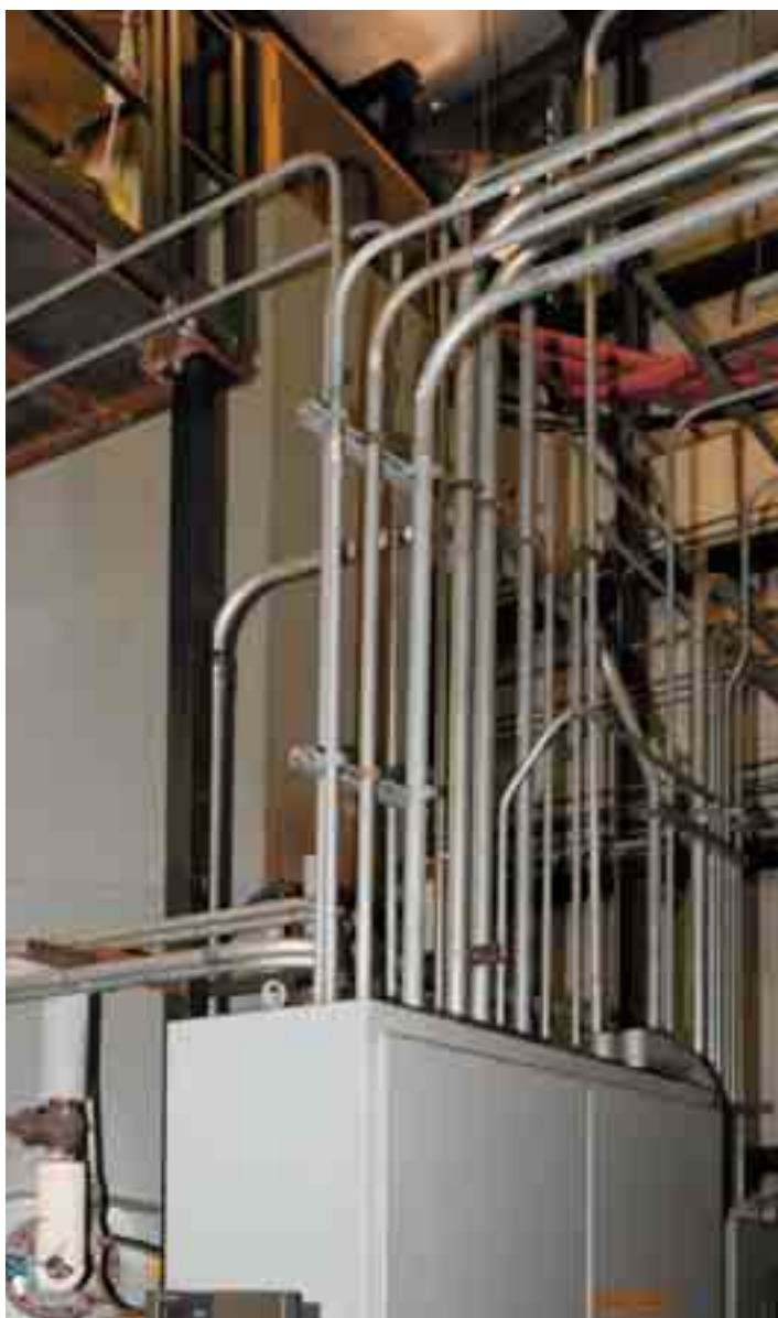
The mill's 33 MW electric boiler runs at off-peak time, is 99.9 percent efficient, and paid for itself in about six to eight months.
