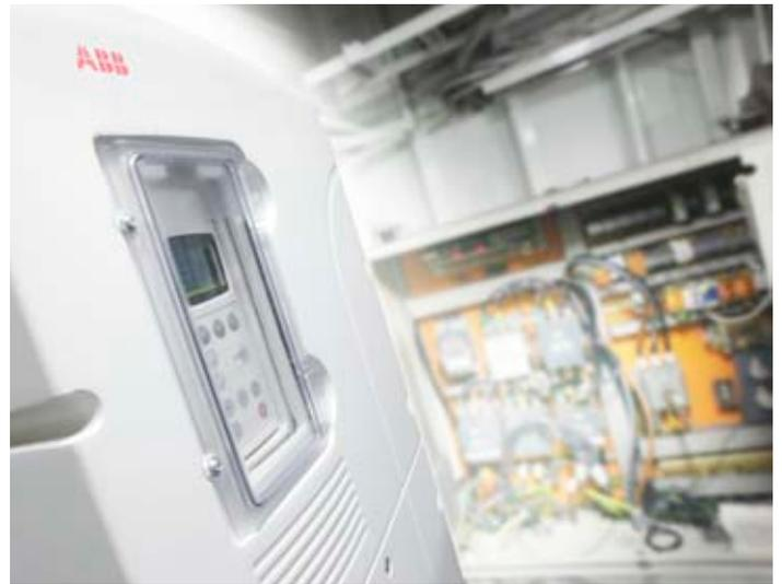
The wall mounted ACS800 industrial drive with built-in winch control program replaced contactors for smooth, trouble free starting.
