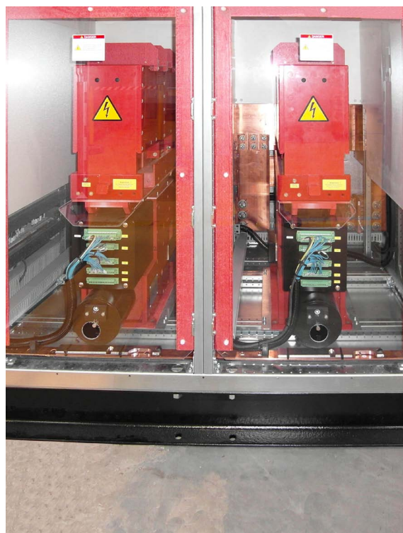
Parallel breaker arrangement
