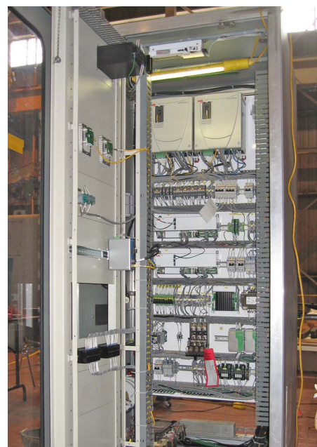
UNITROL M after the control upgrade with the latest UNITROL 6080 control unit
