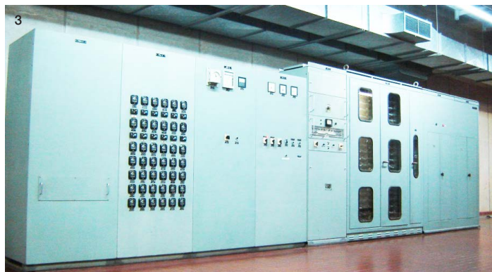
1 Salto Grande hydro power plant | 2 Commissioning group from ABB with engineers and technicians from Salto Grande | 3 Old excitation system from another supplier | 4 ABB UNITROL 5000 excitation system
