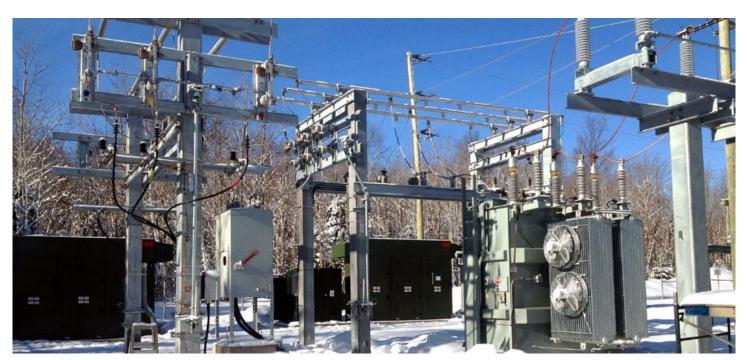
VArPro STATCOM installation at a substation in the Canadian Maritimes to support a growing wind farm installation
