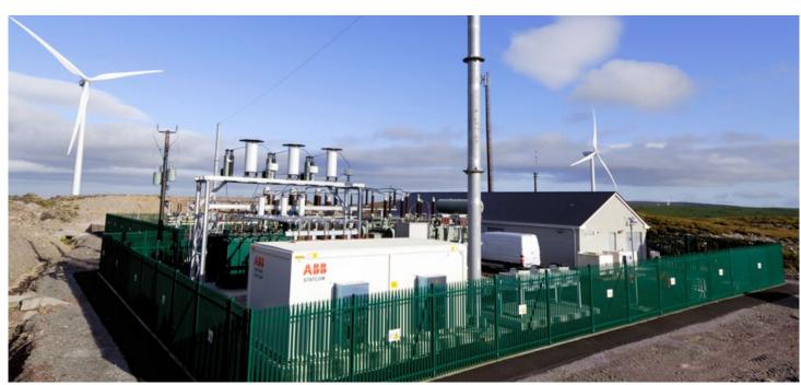
The ABB VArPro STATCOM system, installed at a wind farm in the UK to ensure grid code compliance.
