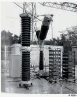
Fig. 2. Design of the breaking unit for HVDC circuit-breaker.
