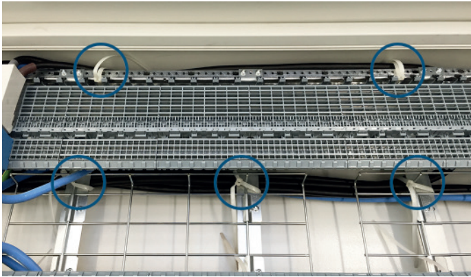
Fig.14: Fixing position of the cables
