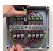
Figure 2: Removing a Lightning Barrier after installation
