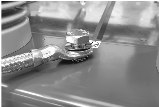
— 47a Tighten the earthing link to the frame of switch-disconnector with torque 40 Nm. Between link's head and switch-disconnector frame must be only toothed washer (excluding frames dedicated to Czech market, where toothed washer is not applicable). Rest of washers must be above link's head
