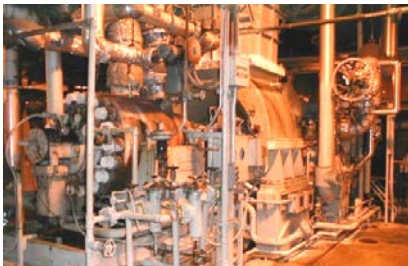
Auxiliary Steam Turbines
