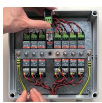
Figure 2: Removing a SPD after installation
