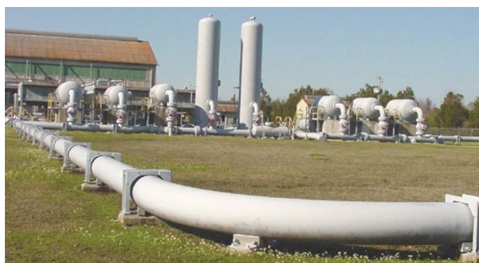
Typical compressor station with scrubber plant
