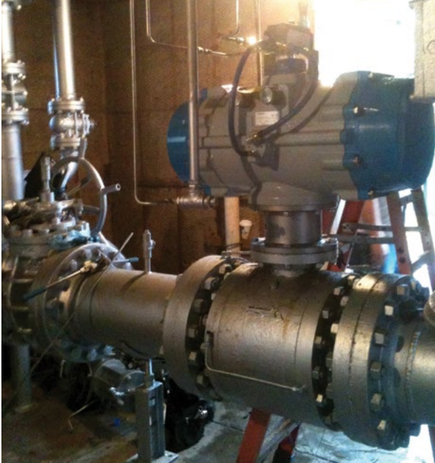
TZIDC positioner shown on rotary actuator
