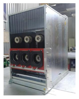
Fig. 6 Retrofill frame with integrated current sensors
