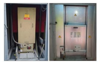
Figure 8. Retrofill of an air magnetic breaker (original at left)
