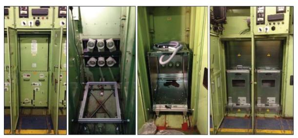
Fig. 5 Retrofill installation sequence
