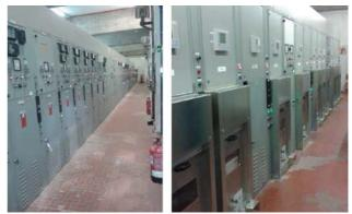
Figure 11. Original switchgear lineup (left) and after retrofill and P&C renewal
