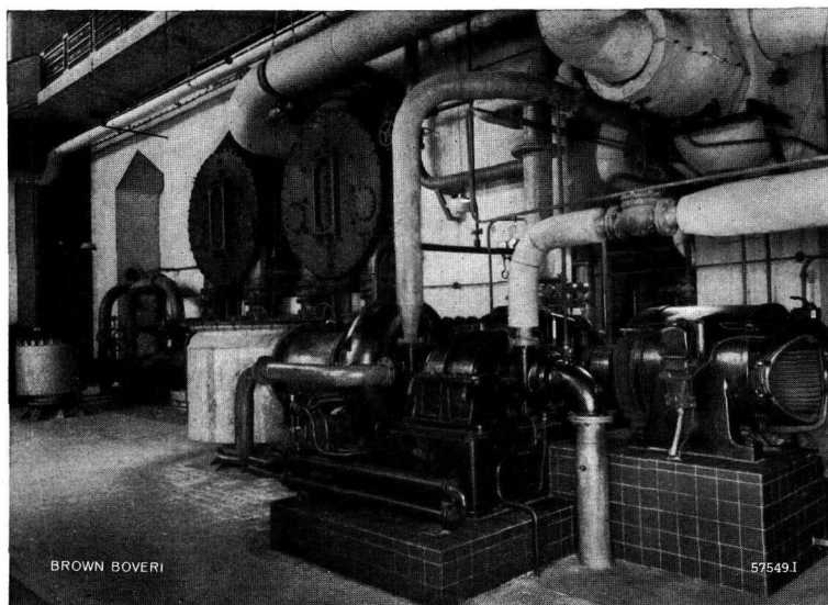
Fig. 9. — Condensers and condenser auxiliaries of a 30,000 kW turbo-set.
