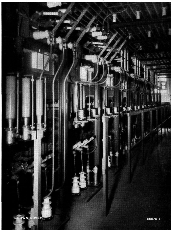
Fig. 40. — Rear view, Fig. 41. — Front view of air-blast high-speed circuit-breaker of 16 kV switchgear.
