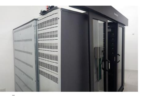
The cabinet planning and implementation included a 3D model, which was presented to the client in order to show how the cabinet would fit into the current configuration and the look of the final installation. It also made installing the UPS simpler once the components arrived on site, as the technicians already had a 3D model to work from.
