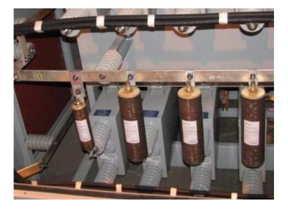
Two-fuse approach for protecting overhead capacitor bank
